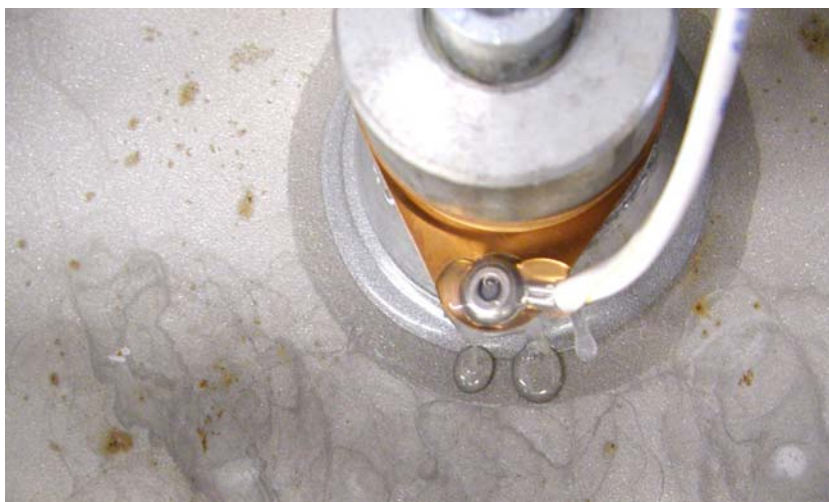
Illustration 11.2. Leaking tank floor with traces of liquid
